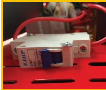
Figure 18 – Circuit breaker
